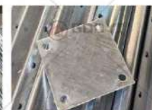
Lacing Bar Board Use at outer of the water tank, to connect the inner lacing bar from outer of water tank.
